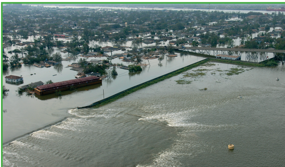
Aerial view of some of the damage related to Hurricane Katrina the day after the hurricane hit- August 29, 2005. This is the levee that has been damaged by the hurricane storm surge.
